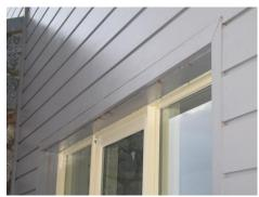
We have recently been working through the Bushfire Hazard Assessment and to achieve the required Bushfire Attack Level of BAL 40 we need to remove all the existing high maintenance and potentially flammable external timber wall cladding and replace with Colourbond Steel Cladding to improve the aesthetics of the building and reduce the fire damage risk at the same time.
